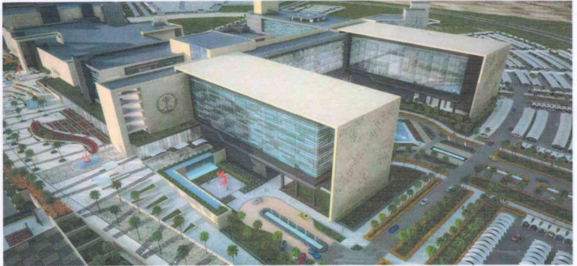
AERIAL VIEW OF MEDICAL CENTER - PATIENT TOWERS AND VIP ENTRY
